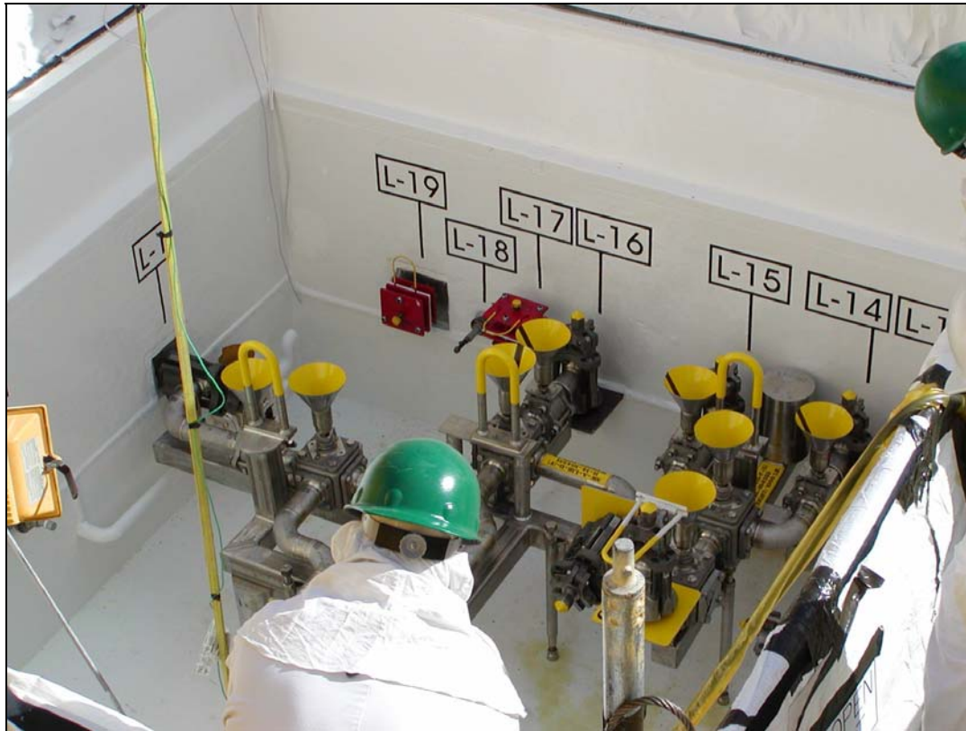
Fig. 3 Transfer Pit Before and After Restorations and Upgrades
