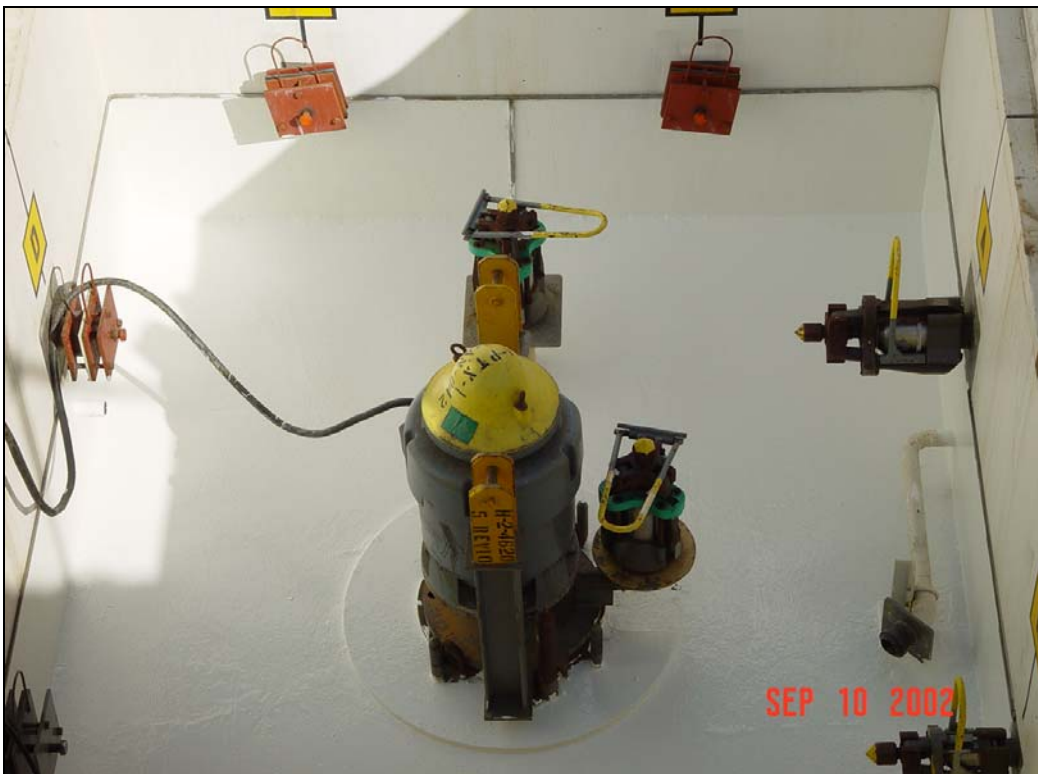
Fig. 4, Tank Pump Pit Before and After Restorations and Upgrades
