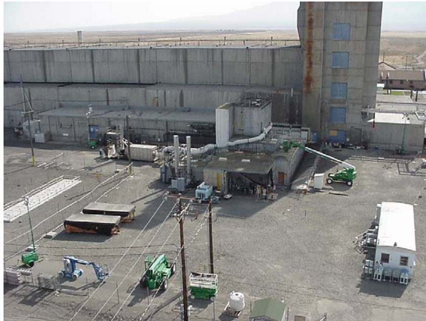
Fig. 1 233-S Facility (photo, looking south, taken before demolition began in October 2003). The 202-S REDOX facility is the large canyon building in background.
