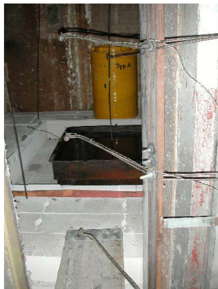
Fig. 1 View through the front door
