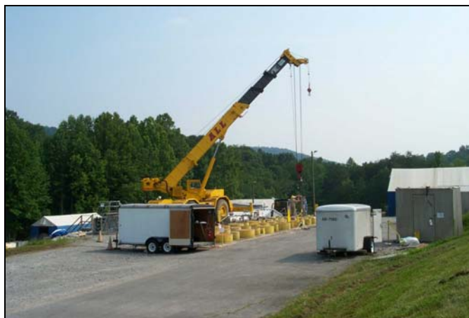
Fig. 2 Crane placement between storage and loading facilities
