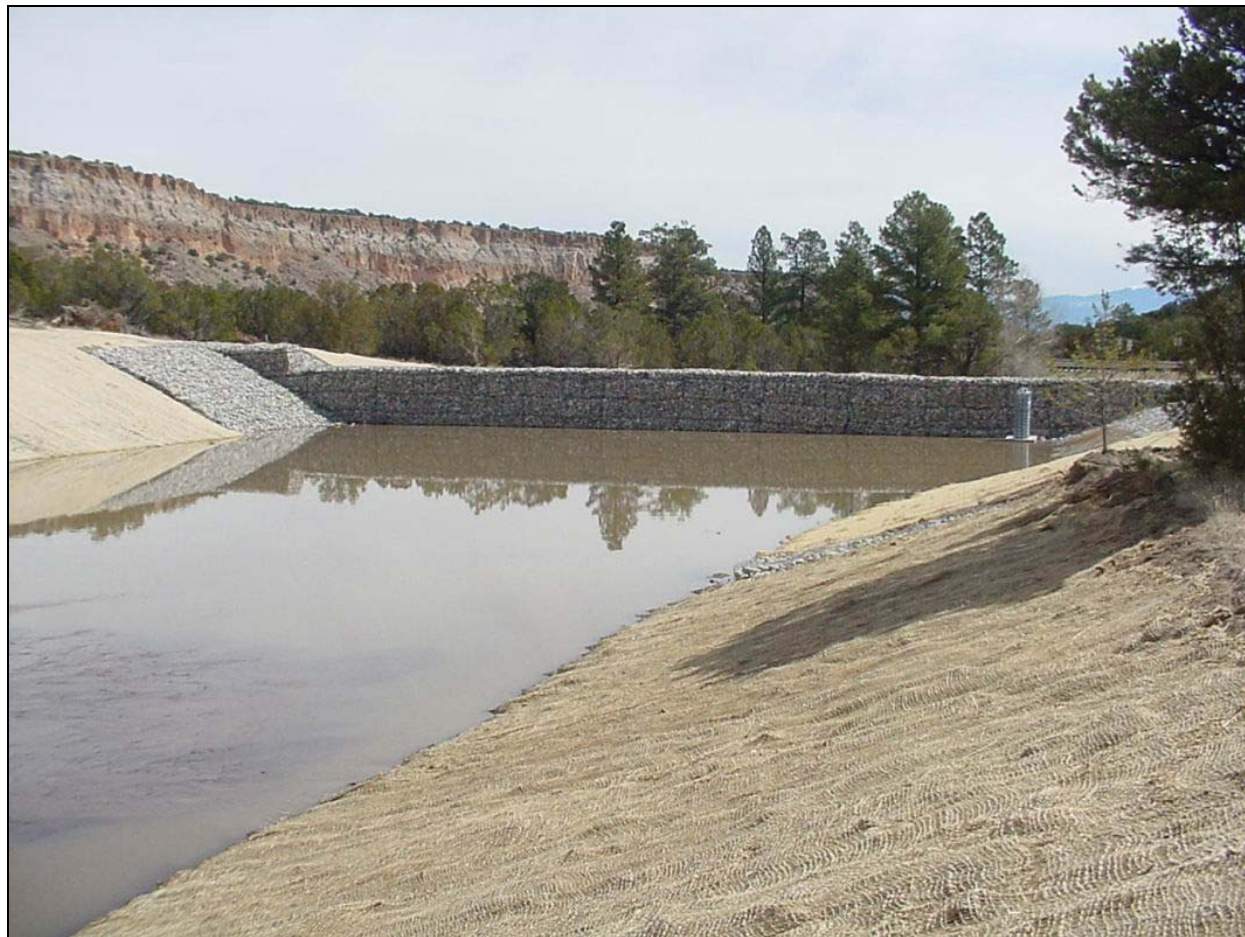
Fig. 1 Photograph of the Los Alamos Canyon low-head weir with ponded runoff
