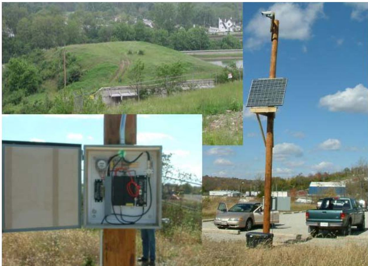
Fig. 2 Machine vision system monitoring the waste repository cap
