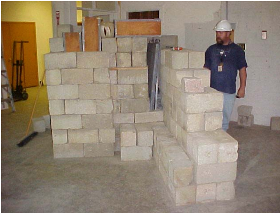
Fig. 3 Martin Latta (Decommissioning Foreman) evaluates unexpected condition (lead plates).
