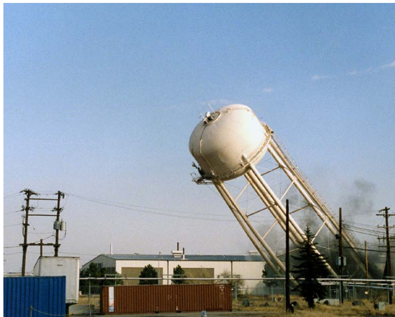
Fig. 4 The Rocky Flats Water Tower was demolished in November
