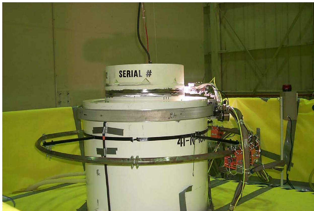
Fig. 4 Welding equipment mounted on the OD of the Sshielding insert while welding an RH-TRU waste container.
