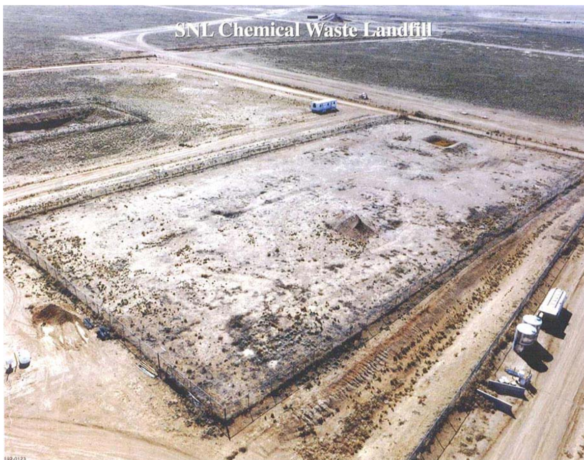
Fig. 2. Chemical Waste Landfill in 1992 (View to the Southeast).
