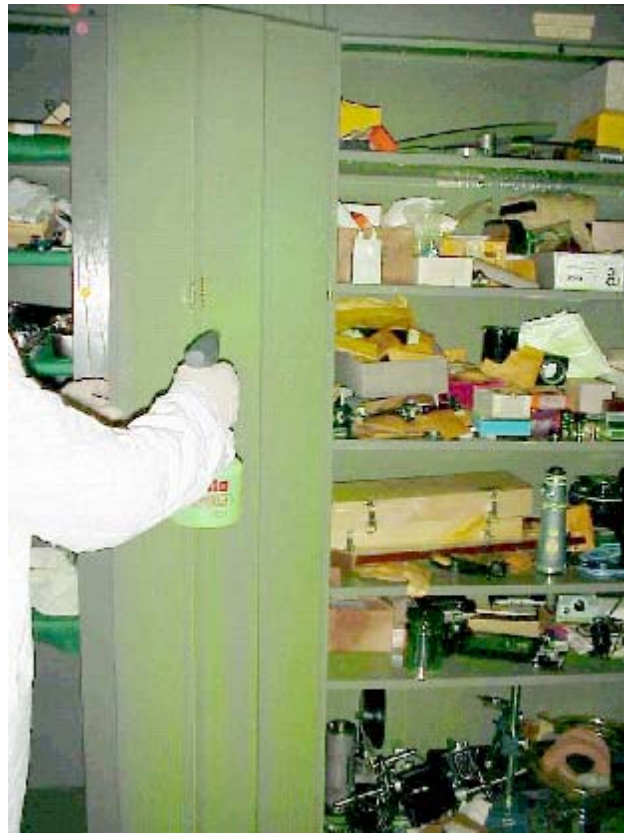
Spray Bottle applying CC Wet to Be/Uranium contaminated materials prior to removal from cabinet.
