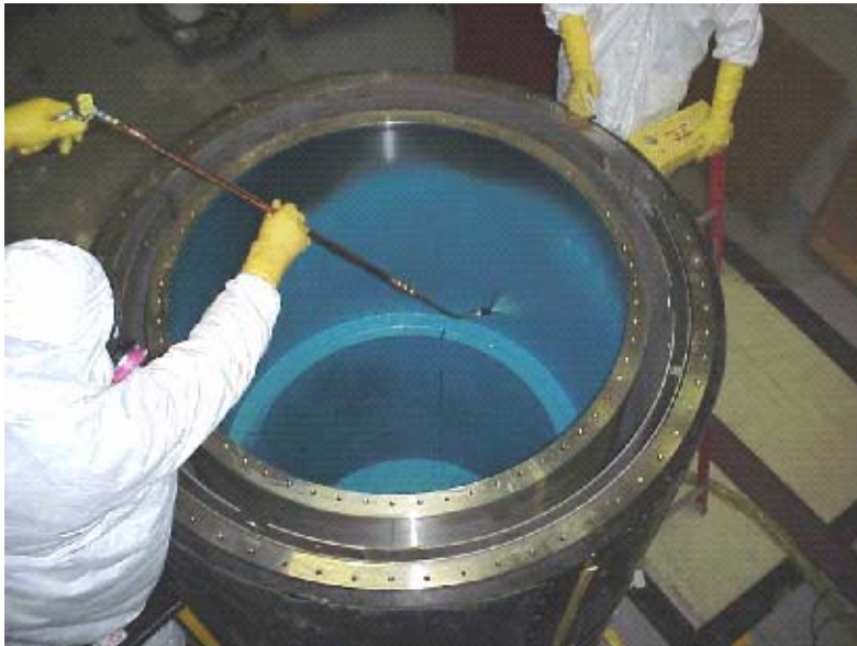
FIX applied to annular tank, B886
