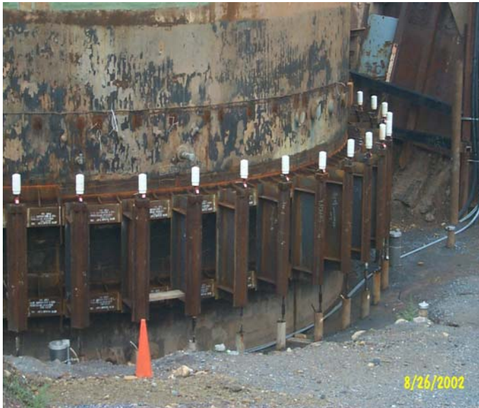
Fig. 3 Anchor and stiffening ring
