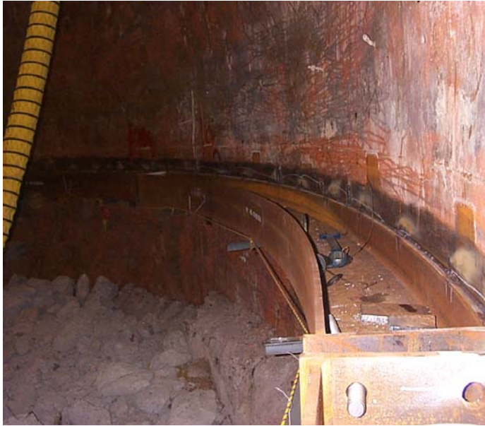
Fig. 4 Anti-Buckling stiffener ring
