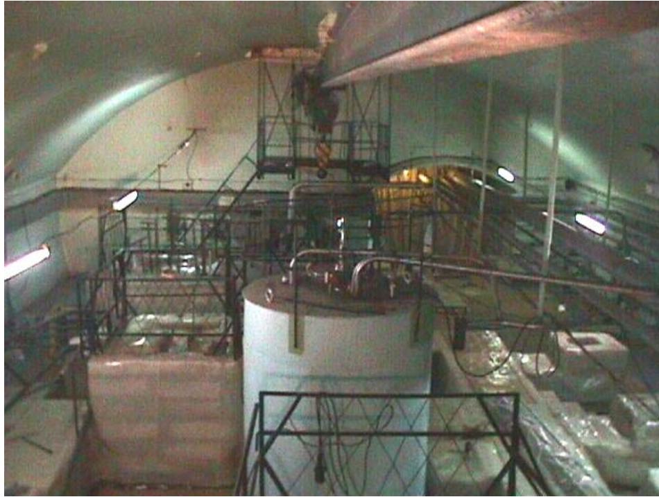
Fig. 4 Support equipment above 3200 m 3 tank being retrieved at MCC
