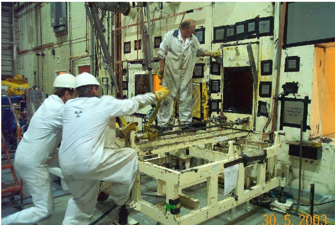
Fig. 2. Removal of Concrete Shield Plug from Wing Wall Interspace.
