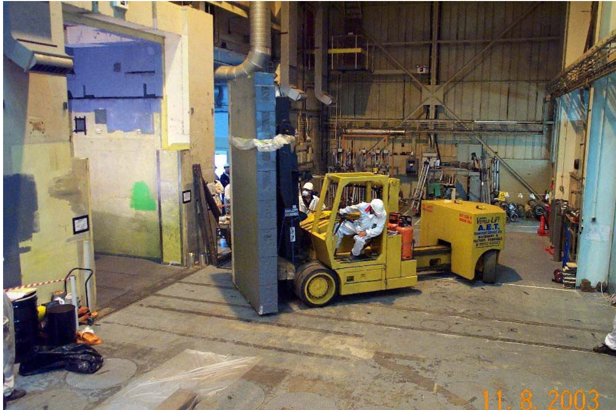
Fig. 3. Removal of Wing Wall with Versalift Truck showing Rear Extension.
