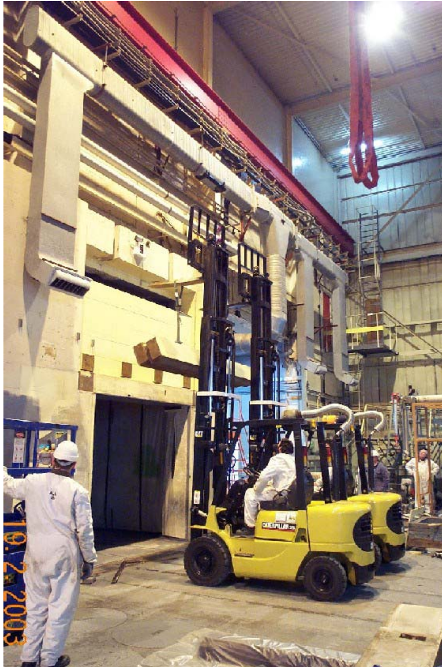
Fig. 1. Trucks Removing Cave 7 Shielding Lintels in Tandem.
