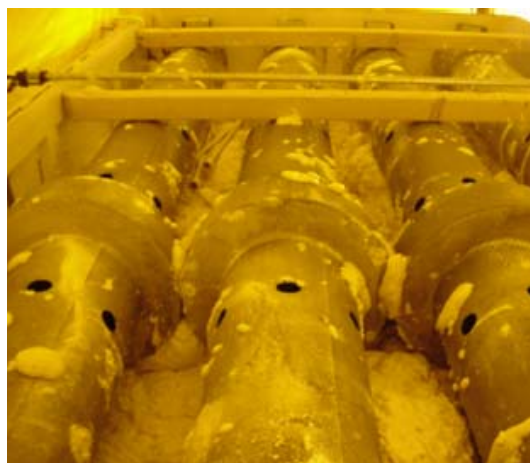
Fig. 3 SP-149 after the application of foam.
