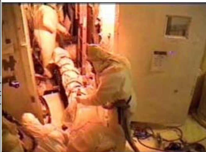
Fig. 4 Removing contaminated process vessel through PPC-S doorway
