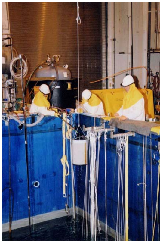
Fig. 2. Removing Used Filters From the FSP for Packaging.
