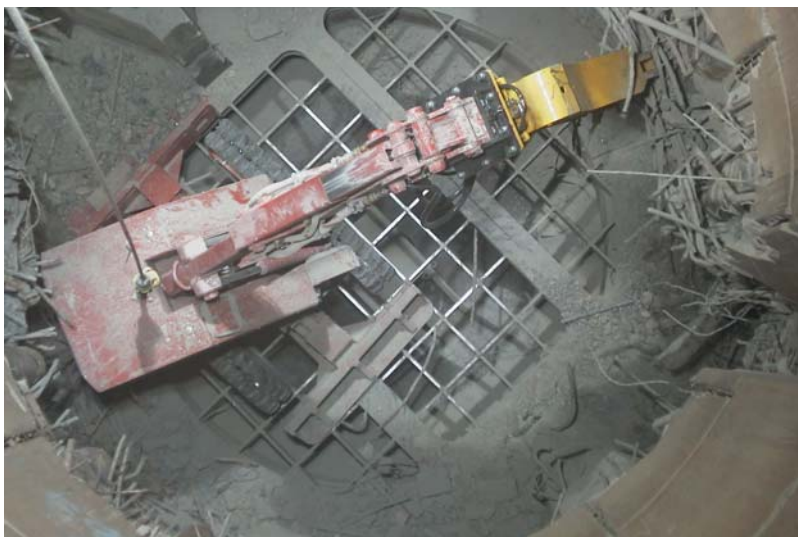
Fig. 2 Excavator I inside the reactor cavity
