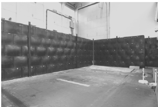
Internal View of North and East Walls
