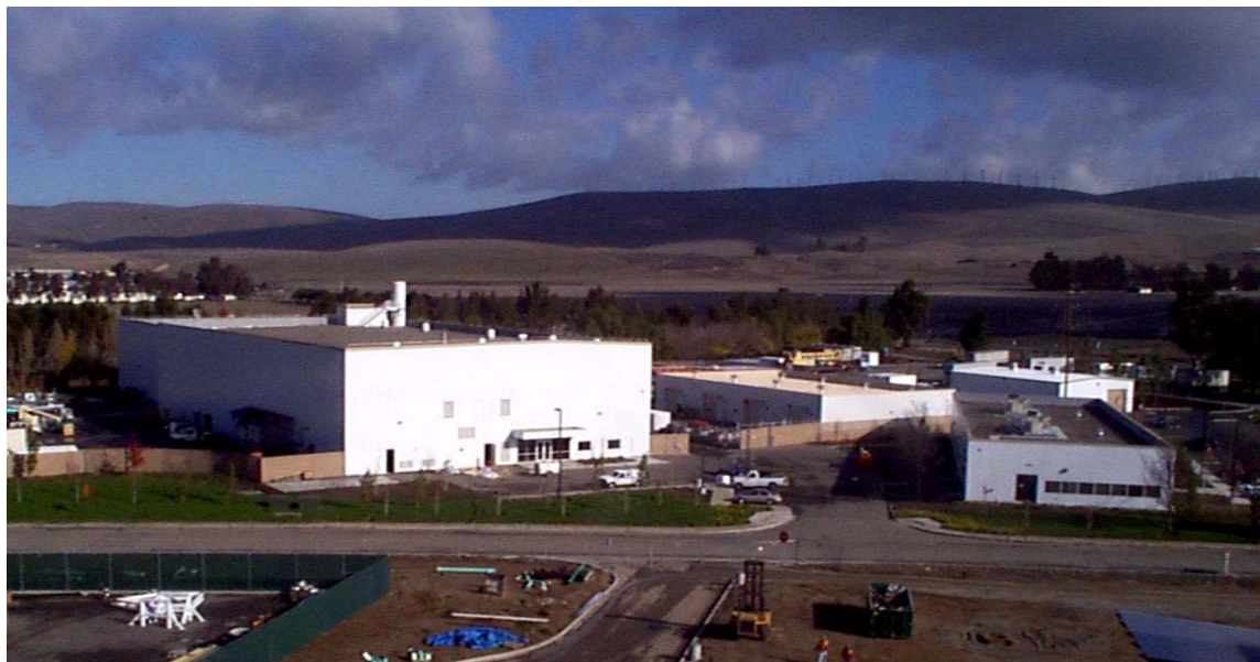
Fig. 1 An aerial photo of the decontamination and waste treatment facility (DWTF)
