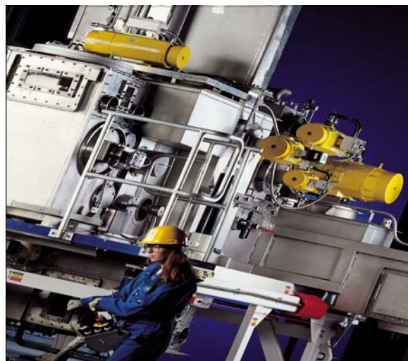
Fig, 1. Retrieval & Remediation Operations at Sellafield.
