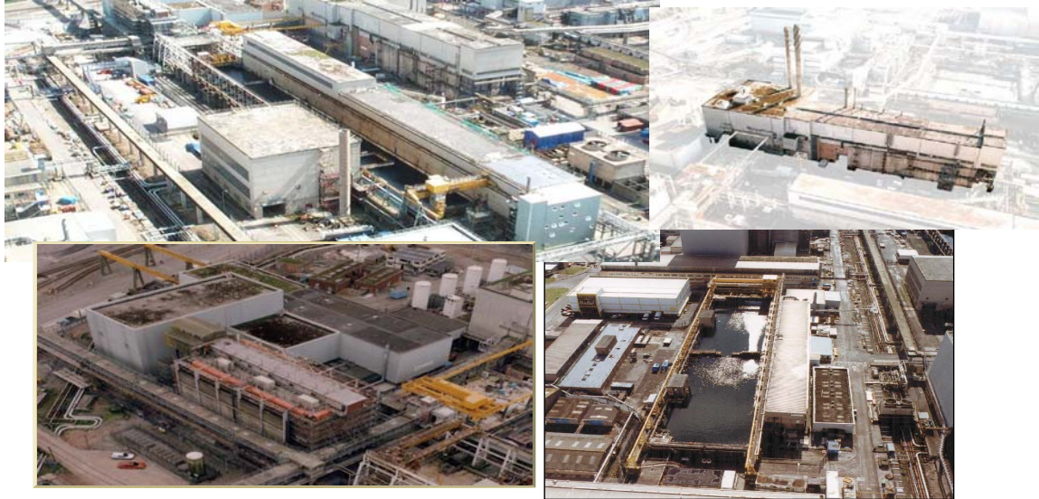
Fig. 5 “Legacy ponds & silos containing intermediate level solid, liquid and corrosion product sludges”
