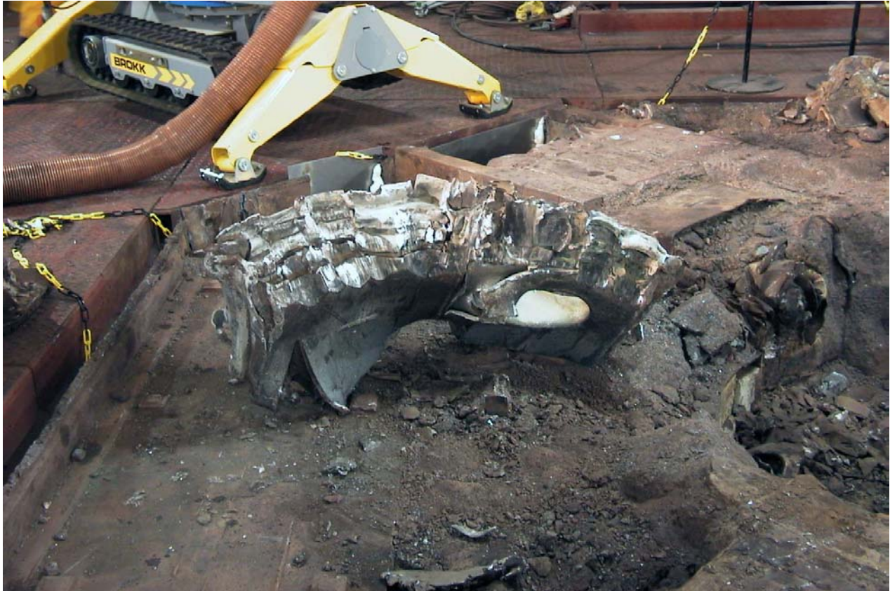
Fig. 4 Part of the Thermal shield separated by the rock chisel
