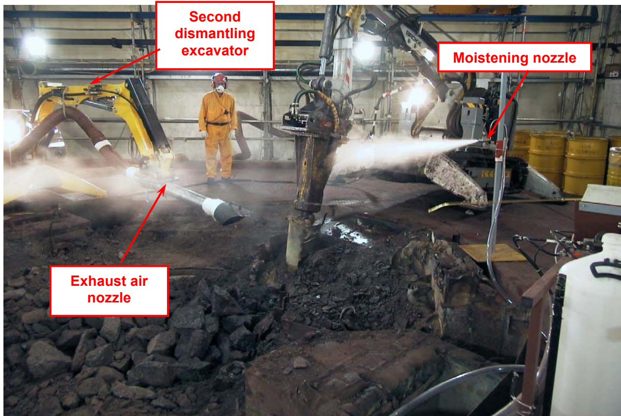
Fig. 3 Moistening and air extraction during operation of the rock chisel
