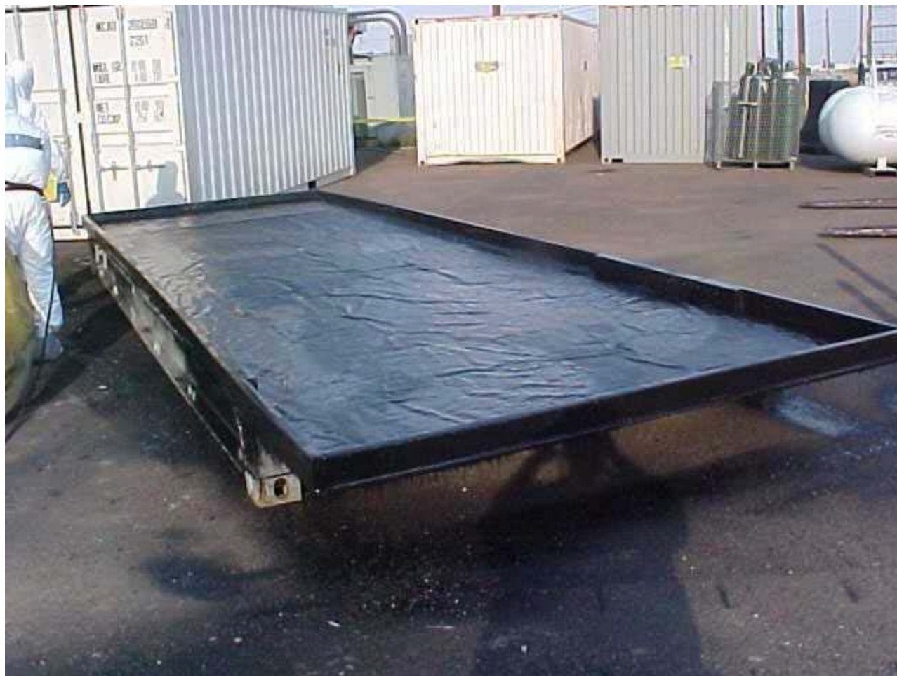
Fig. 3 Completed base ready to accept the waste item
