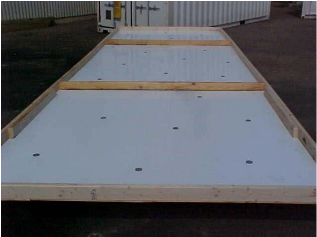
Fig. 2 Base constructed to accept the footprint of the waste item
