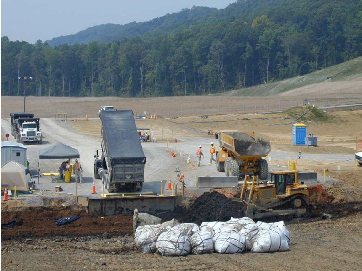
Figure 1. Waste Placement at the Lower Dump Ramp in the EMWMF Disposal Cell
