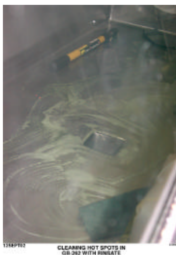
Figure 2. Decontamination of a LANL glovebox using EAI Technology
