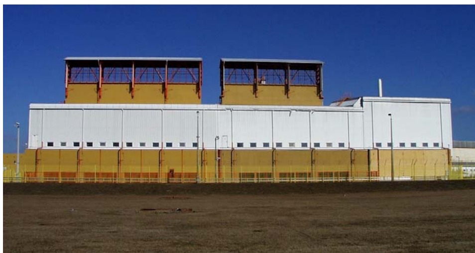
Fig. 3. Paks MVDS – shown in 2000 after first extension vaults were added
