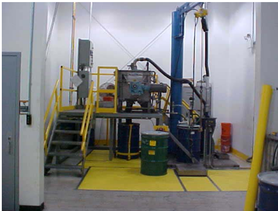
Fig. 1. Elemental mercury stabilization process at M&EC
