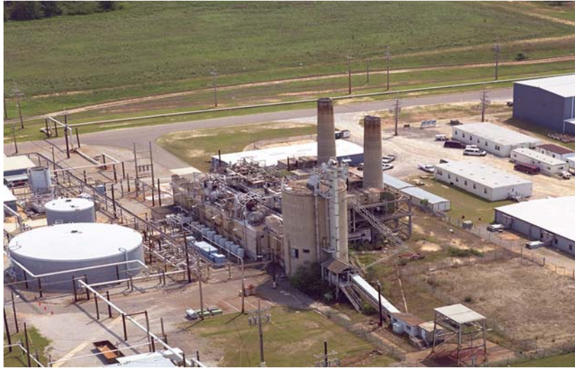
Fig. 2. Assets for Services Program – F-Area Powerhouse (Before Demolition)
