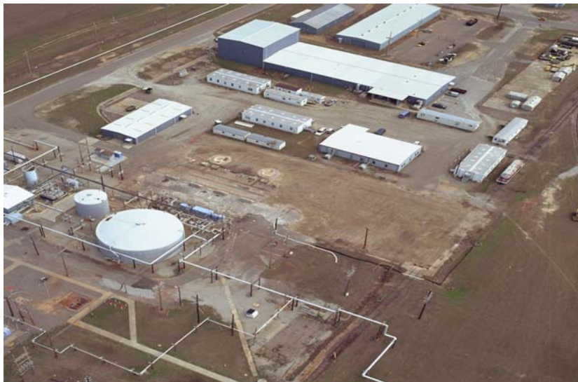
Fig. 3. Assets for Services Program – F-Area Powerhouse (After Demolition)
