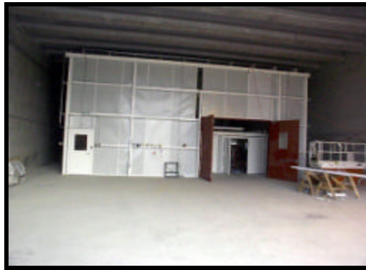
Fig. 1. Waste Sort Facility (WSF)
