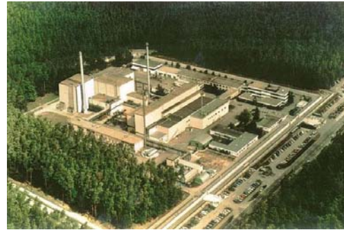
Fig. 1 Aerial view of the WAK Karlsruhe
