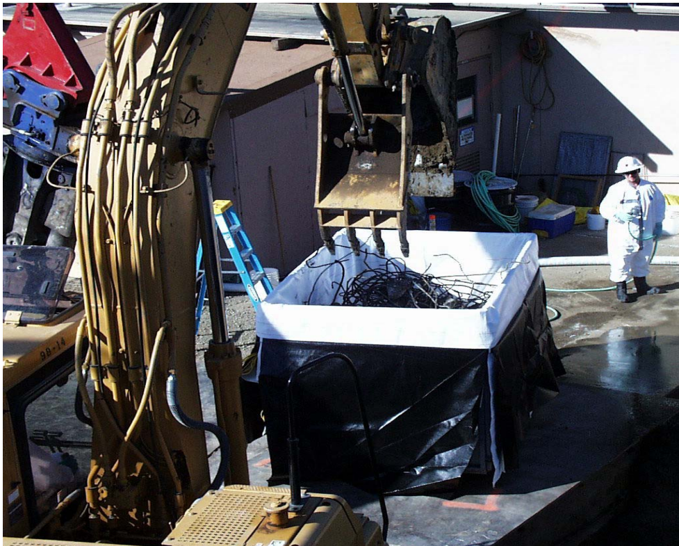
Fig. 4. Excavator Loading Debris into 7.0 Cubic Meter (9.1 Cubic Yard) Lift Liner®
