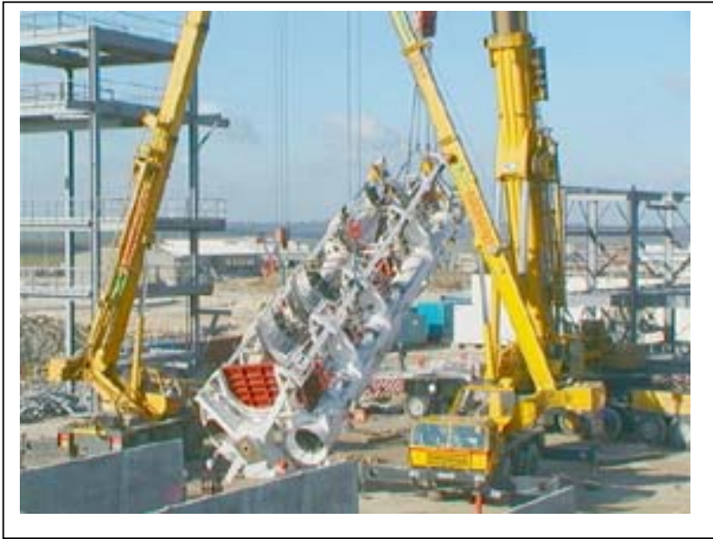
Fig. 4 - Assembling of the sinking platform
