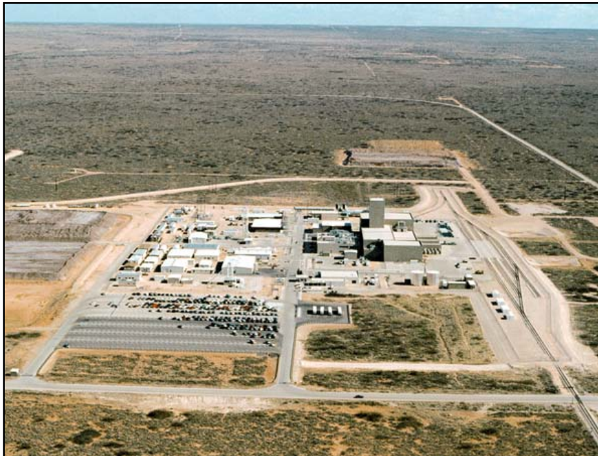
Fig. 2. Aerial view of the WIPP site
