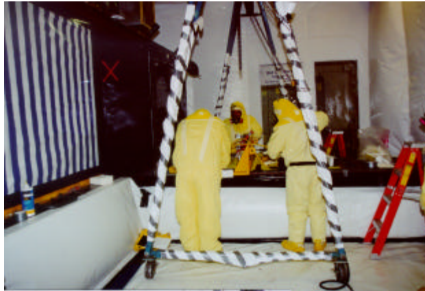
Fig. 1. Shield Window Refurbishment
