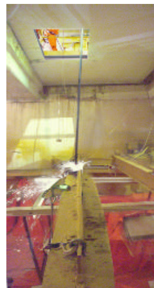
Fig. 3. Oxy-gasoline Cutting of PMC Crane Bridges
