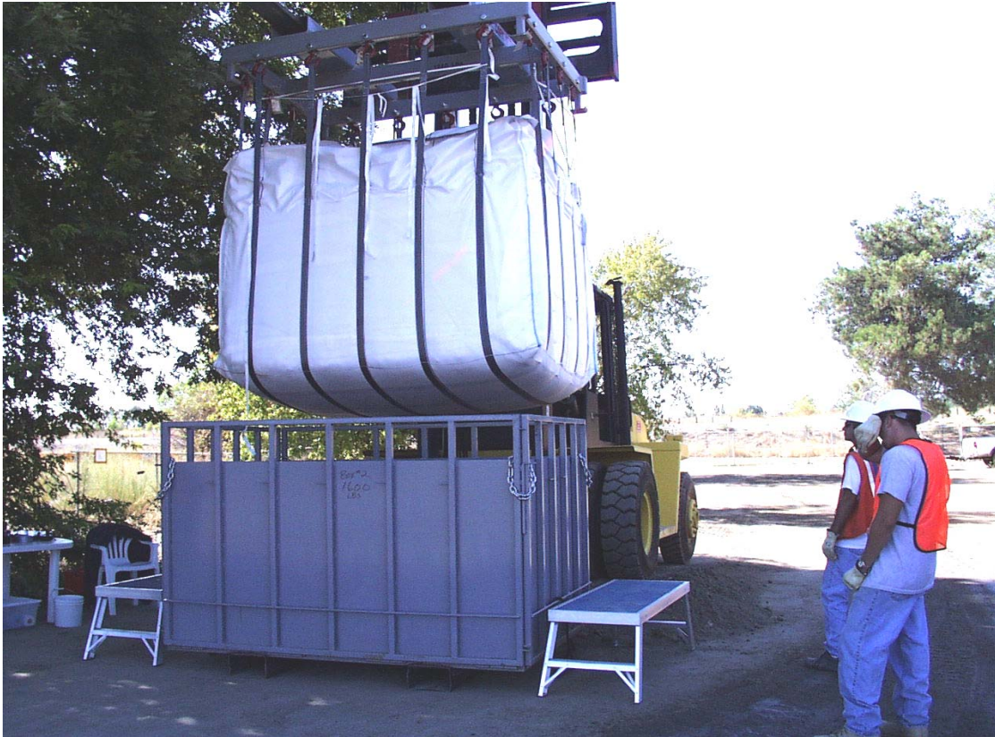
Fig. 4. Removal of 9.1 Cubic Yard Soft-sided Lift Liner® from Loading Frame at the LEHR site
