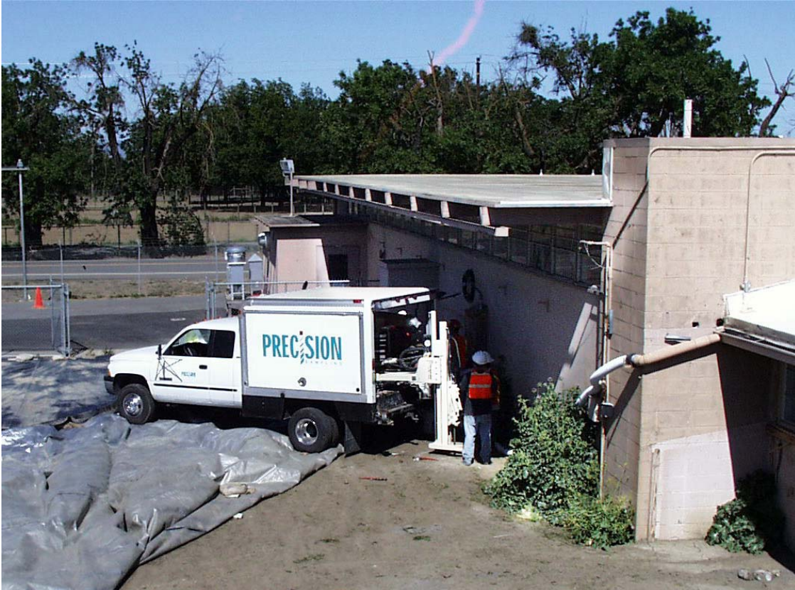
Fig. 3. Direct Push Sample Collection System
