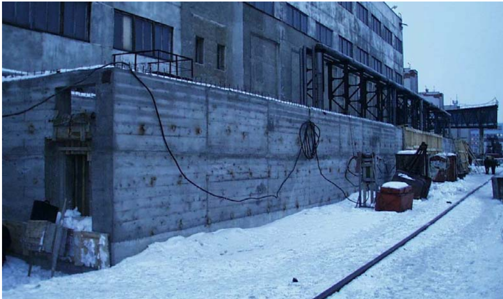
Fig. 4. Construction progress on the AMEC transshipment pad (December 3, 2001).
