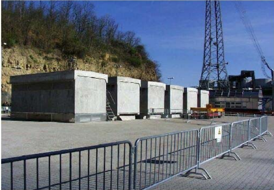
Fig. 3. Interim Storage Area Neckarwestheim
