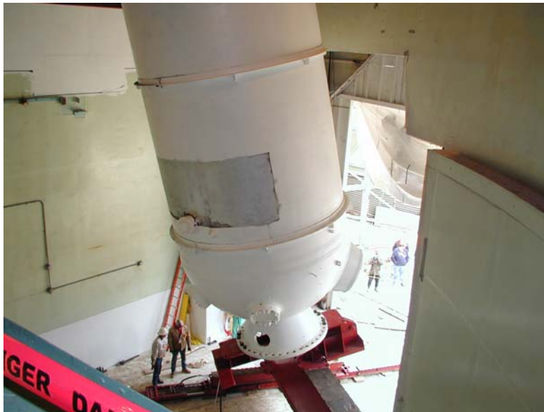
Fig. 1. Steam Generator #1 being down-ended
