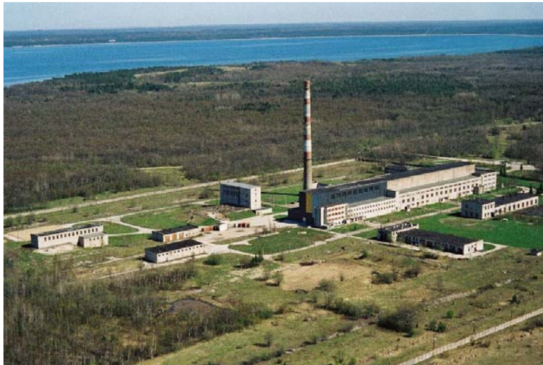
Fig. 1. Paldiski main building (on the right) is sheltering the two Reactors Compartments
