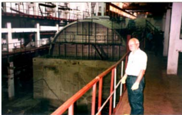
Fig. 2. Erection of the sarcophagus around the reactor Compartment #2, 1995
