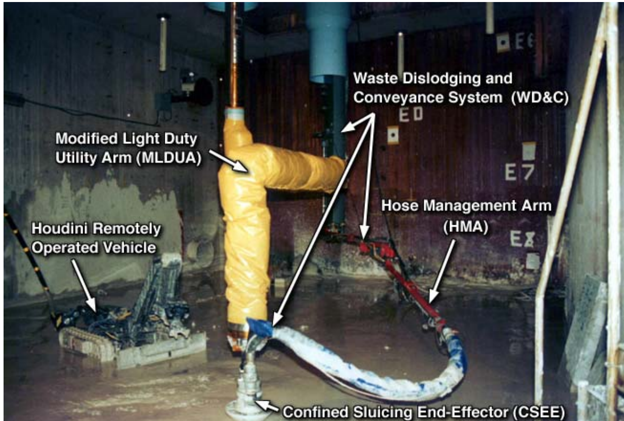
Fig. 3. The primary in-tank components of the Radioactive Tank Cleaning System (RTCS) used during the Gunite Tanks remediation project are identified in the photo above, which was taken during cold tests/demonstration of the technologies.
