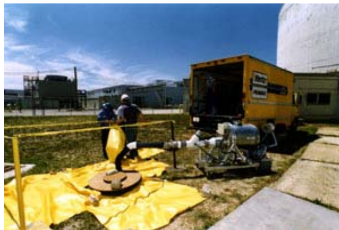
Fig. 2: Pipe Explorer Deployment Setup
