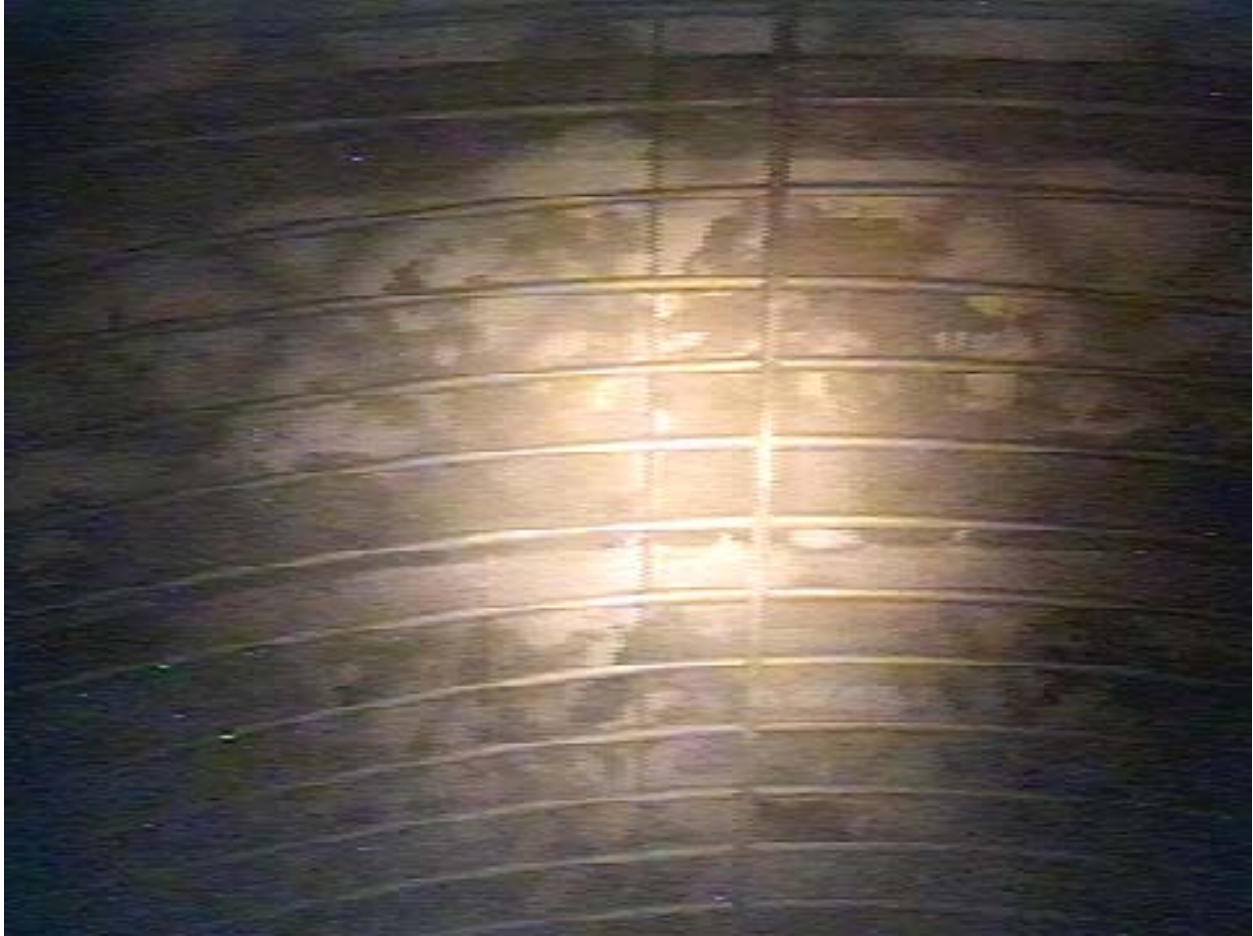
Fig. 4: Tank WM-182 after the October wash ball test.
