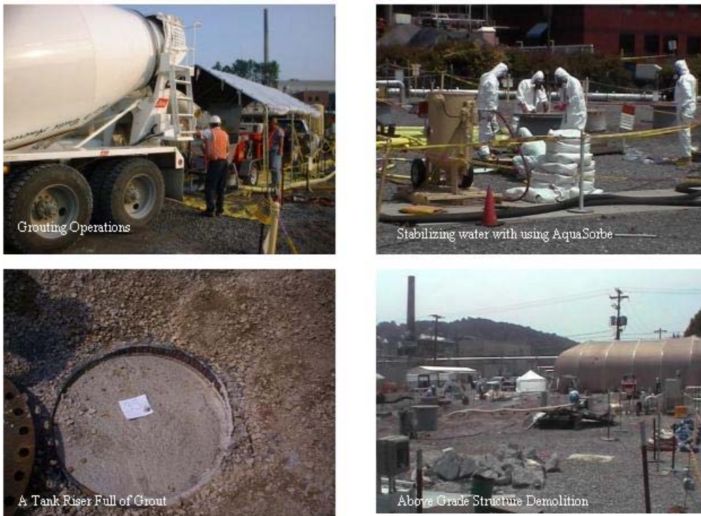
Fig. 2. GAAT Stabilization Field Activities.
