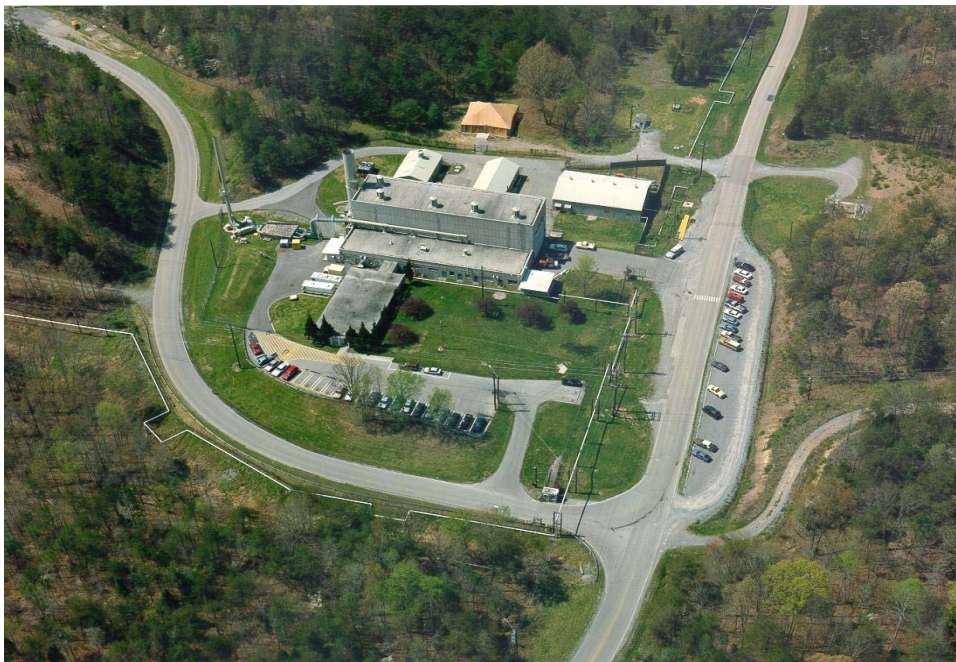
Fig. 1 Aerial view of the MSRE facility
