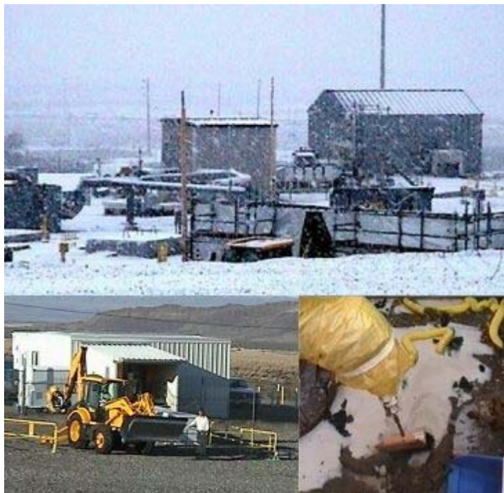
Fig. 1. Pit Viper Deployed at Tank 241-C-104
