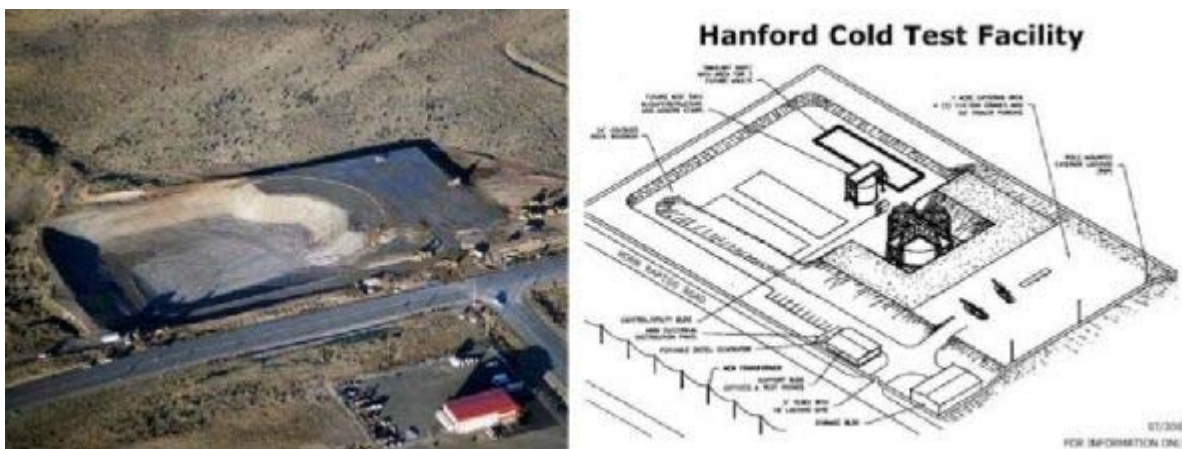
Fig. 4. Hanford Cold Test Facility Construction and Sketch
