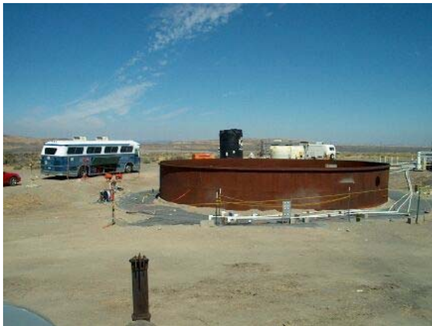
Fig. 3. LDMM Demonstrations at 105-A Mock Tank Leak Site
