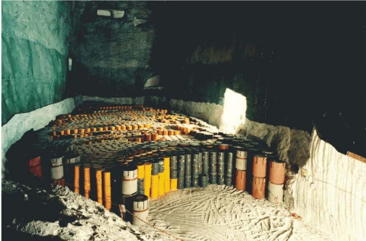
Fig. 2: Deep Geologic Disposal at Morsleben - Eastern Field
