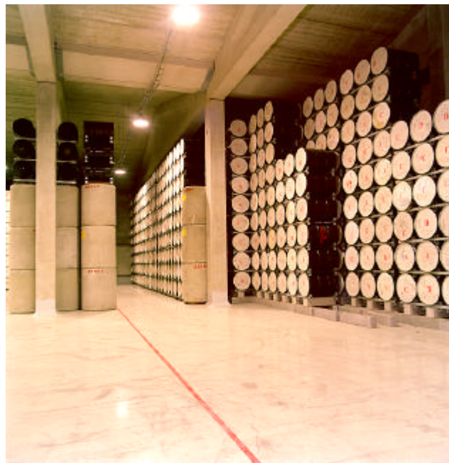
Fig. 2. Storage of low and medium level waste
