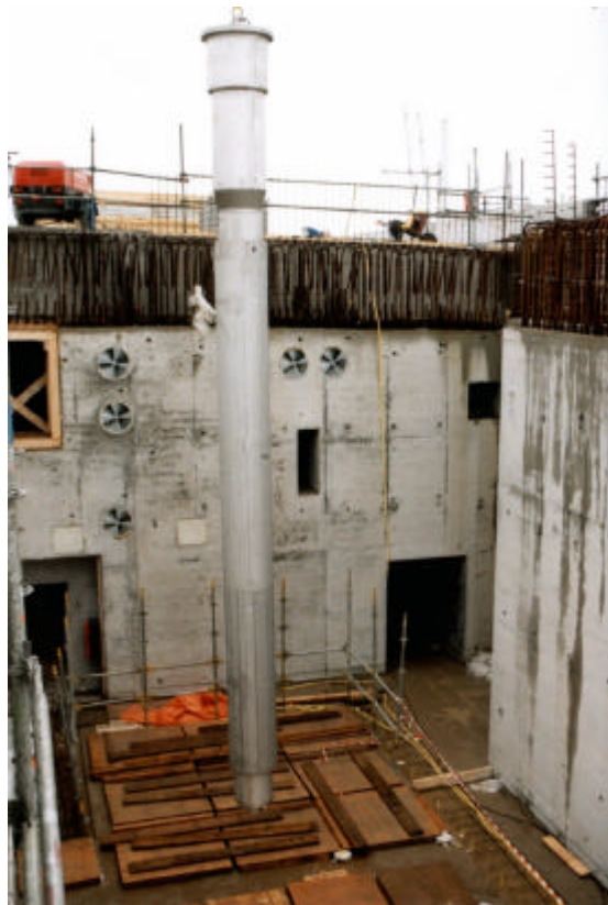
Fig. 4. Emplacement of the wells during construction.
