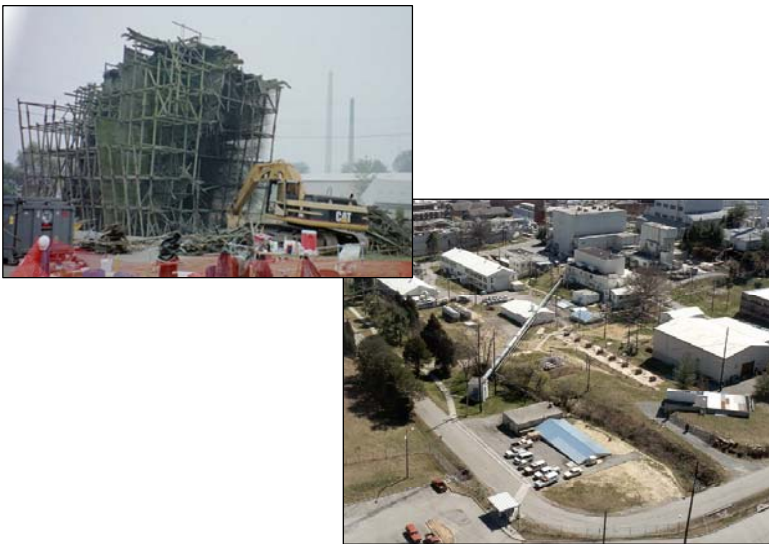
Fig. 3.3. Cooling Towers Demolition.
