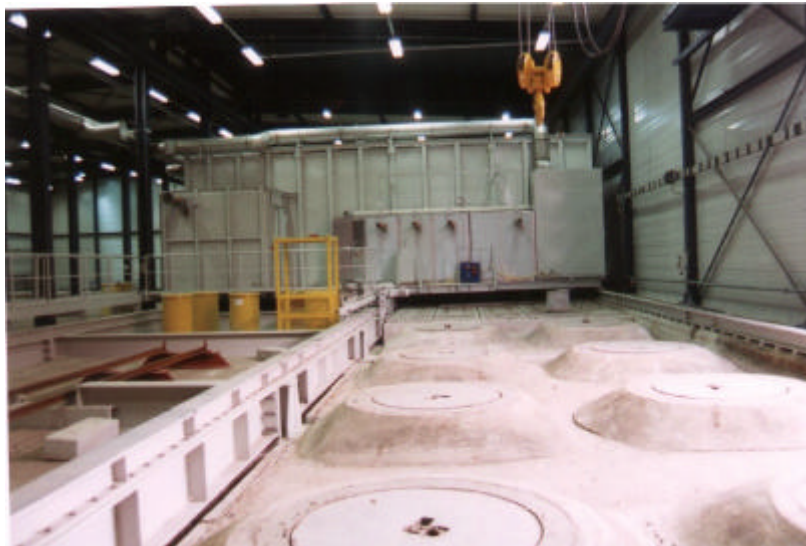
Fig. 4: Caisson on the rail carrier construction
