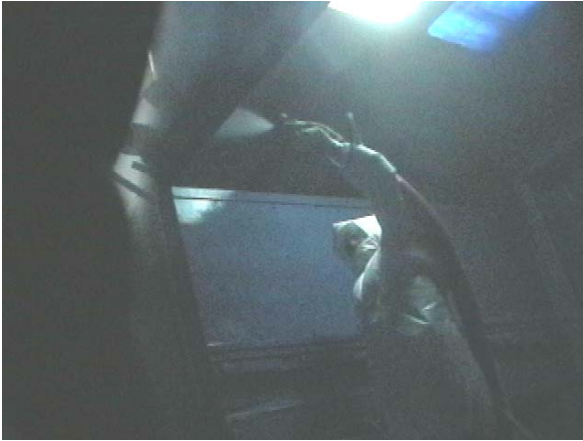
Fig. 1. Instacote installation in PermaCon
